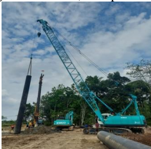
Gambar.9 Temporary Casing
