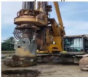
Gambar. 2 Pekerjaan Pre-boring
