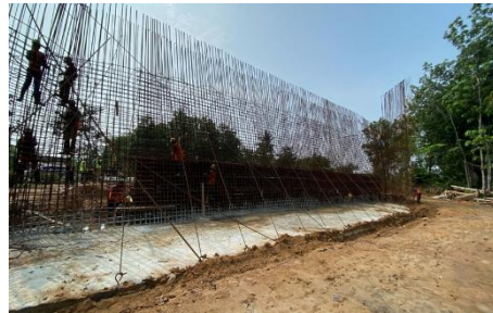
Gambar 16. Pembesian dinding abutment
