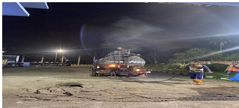
Gambar 2 prime coat
