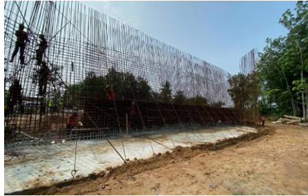
Gambar 16. Pembesian dinding abutment
