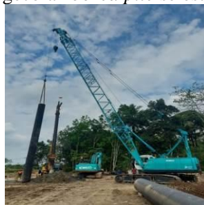
Gambar.9 Temporary Casing
