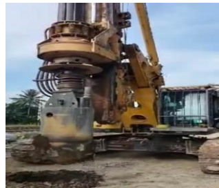
Gambar. 2 Pekerjaan Pre-boring
