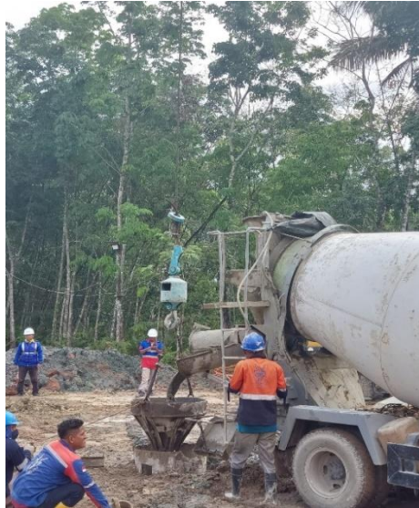
Gambar 2. Pengecoran Bored Pile
