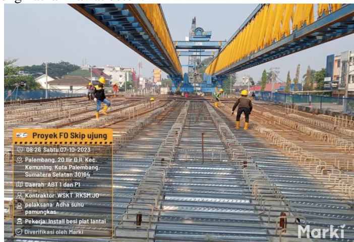
Gambar 2 pembesian deck slab fly over sekop ujung
